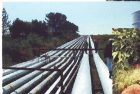
Turnkey based Government's pipeline project
